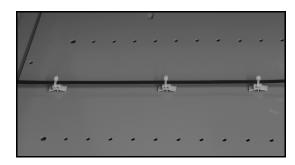
Figure 2.34 Black-Jacketed Fiber installation Example
