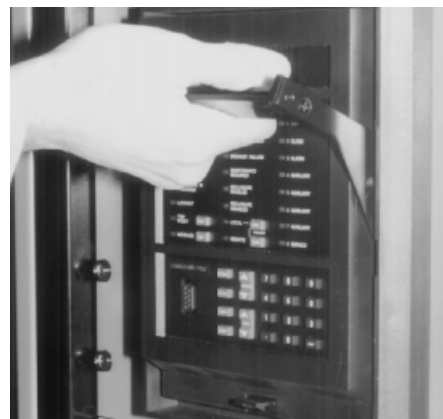
Rotate Handle to Stop Position
