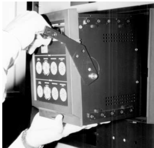
Figure 2-6: RELAY INSERTION
